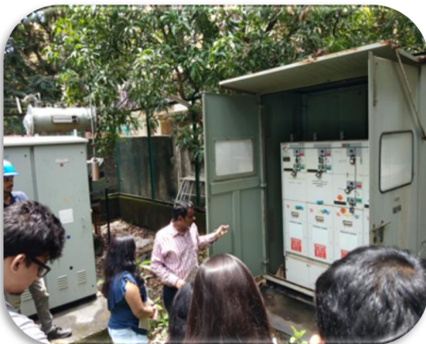
Visit to Sub station
